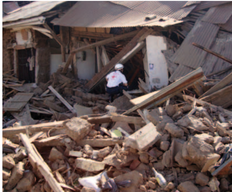
Following the devastating earthquake on 28 February 2010, Chilean Red Cross volunteers carried out emergency response activities such as search and rescue, evacuating patients, removing debris and recovering bodies. Photo: Chilean Red Cross.
